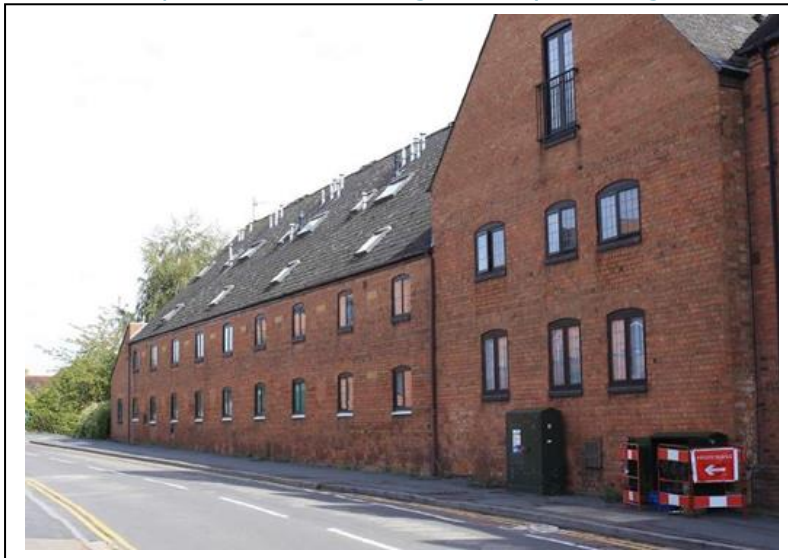
Photo- Clopton Road surviving brewery buildings
